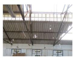
a) Tubular Truss Roofing System for Metal Sheet Roofing
