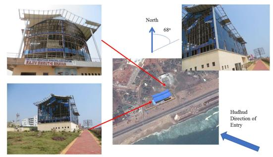
Figure 7: Damaged Gandhi Family Museum in Chinna Waltair Showing Significant Glass Damages in the front and End Sides of the Building
