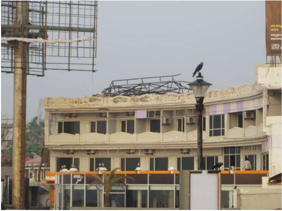
Figure 6: Roof Addition Failure on Beach Road, Vizag.
