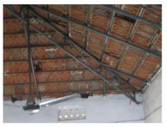
b) Truss and Frame Support for Tile and Shingle Roofing
