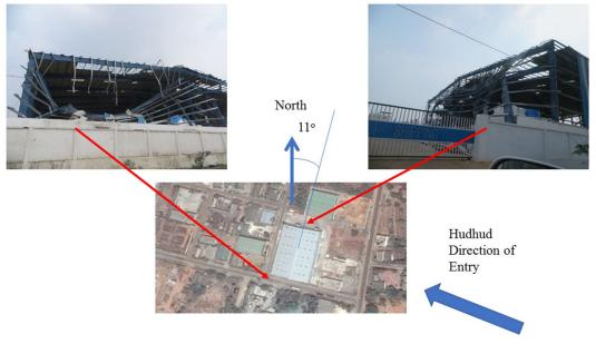
Figure 4: Wind Damaged Steel Storage Structure at 1 Km (3,280 ft) Distance Away in Autonagar, India
