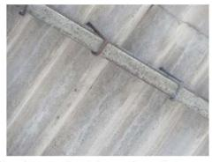
d) Hook Connection of Sheet Metal Roofing
