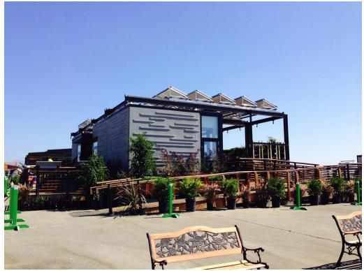
Figure: 2.4 Urban Eden precast geopolymer cement concrete home produced by UNC Charlotte for the 2013 U.S. Dept. Energy Solar Decathlon.
