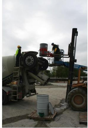
Figure: 2.6 Activating solution pouring into concrete mixing truck.
