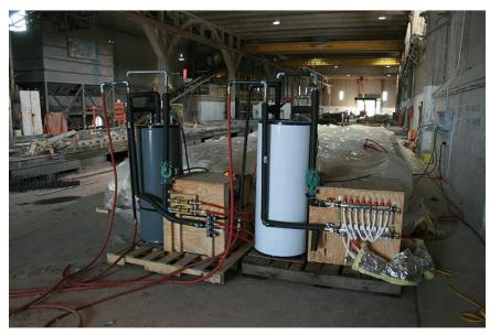
Figure: 2.8 Water heaters set up for heat curing of concrete.
