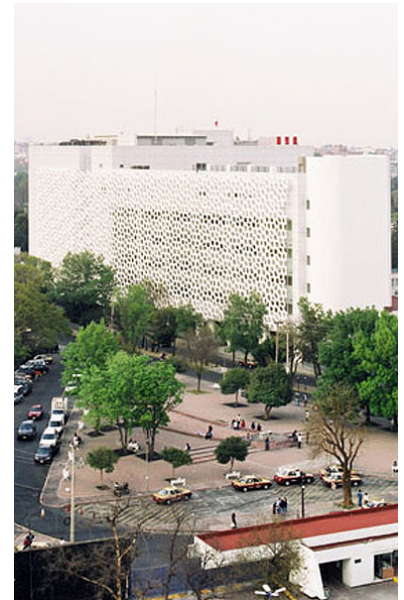
HOSPITAL MANUEL GEA GONZÁLEZ MEXICO CITY, MEXICO
